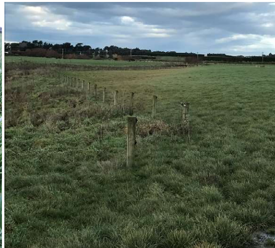
Figure 3: Flood damaged pasture along the creek
