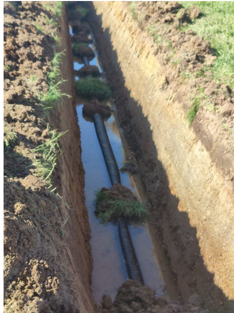
Figure 5: Drainage works at the support block.
